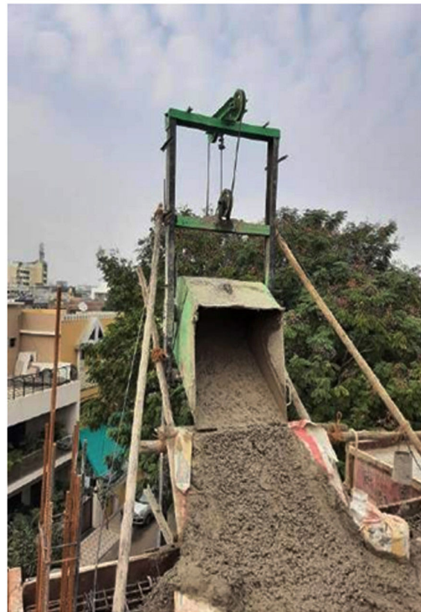
Fig. 4: Fig. of real time elevator with hopper releasing concrete on floor
