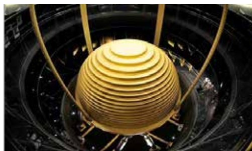
Figure 13 Mechanism of Damping, Taipei 101 Source: www.ctbuh.org/papers
