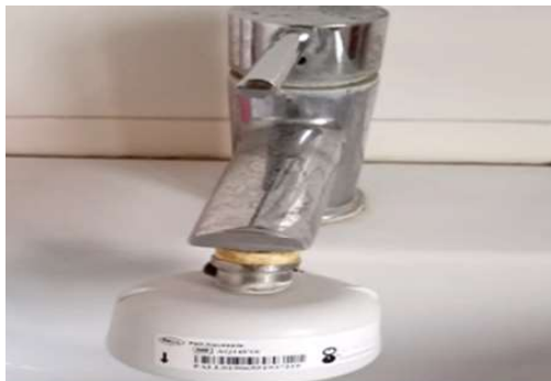
Fig. 6: Pall Aquasafe Water filters installation
